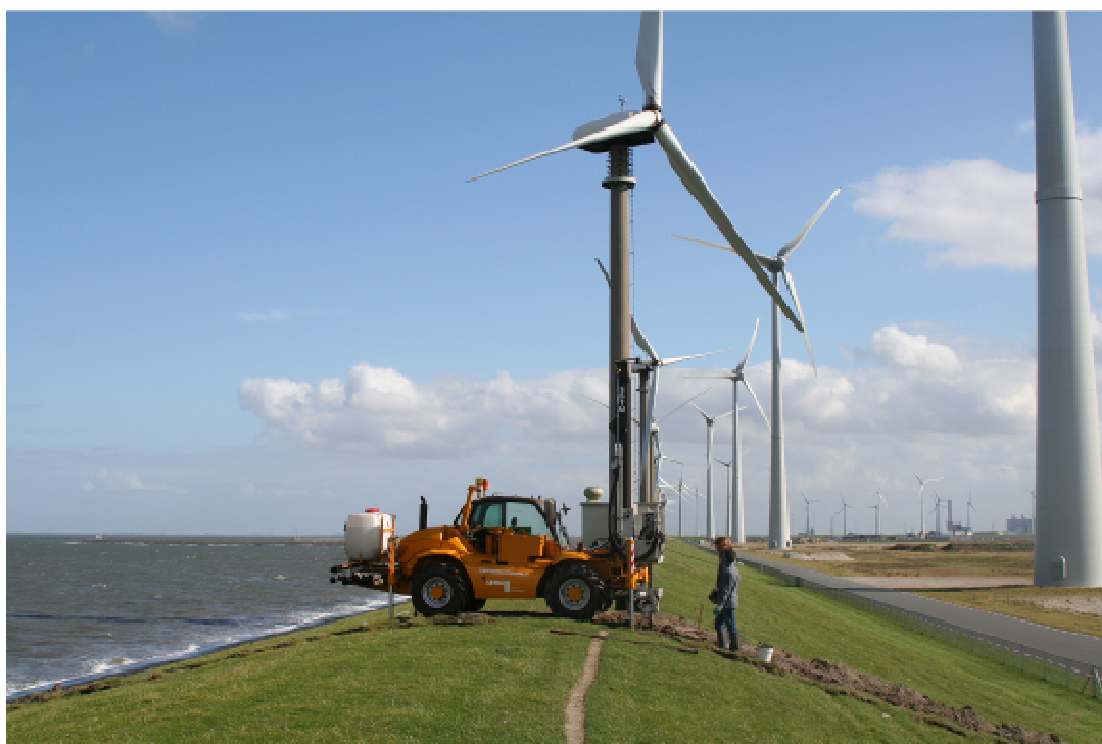
Fig. 2 Installing the sensors
