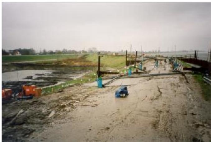
Fig. 8. Dyke failure due to uplift mechanism.
